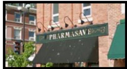
Decorative lighting features enhance architecture
