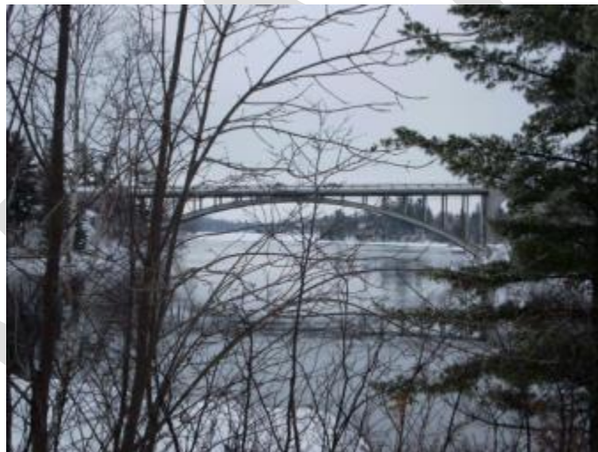
Figure 1: Keewatin Bridge (source: City of Kenora)
