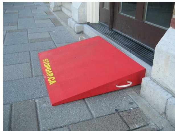
Figure 7 - Customized portable ramps are a simple method to improve accessibility
