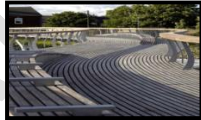
Benches incorporated into bridge design
